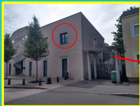
Premises on the top left
