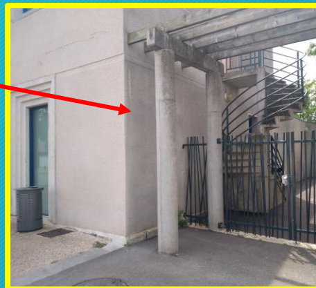
Entrance via the spiral staircase
